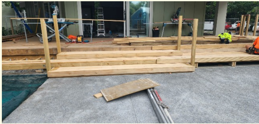
Decking, hand rails, steps and ramp being installed.
